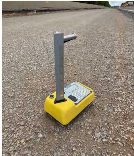
Figure 5: Testing Site 2 – Soil-aggregate reinforced subgrade with nuclear gauge device
