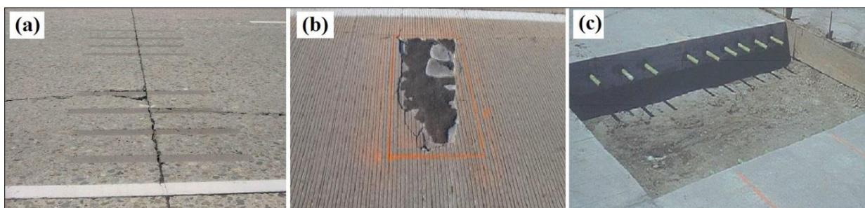
Figure 1. Concrete pavement repair types. a) Dowell retrofit, b) Partial-depth repair, c) Full-depth repair [2], [3]
