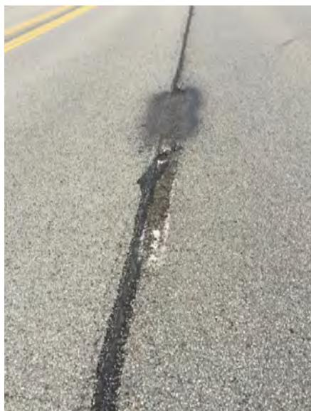
Figure 12: Aggregate pop out and pothole on US 422 skip lines
