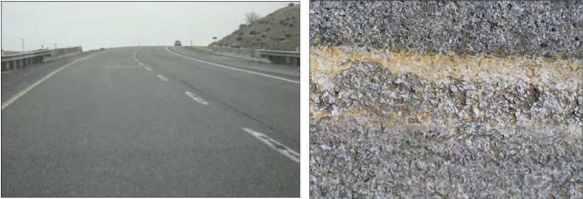
Figure 5: Pavement distress focused in pavement markings taken in Spring 2009 near Santaquin, Utah when the pavement was 6 years old with water based paint markings [18].
