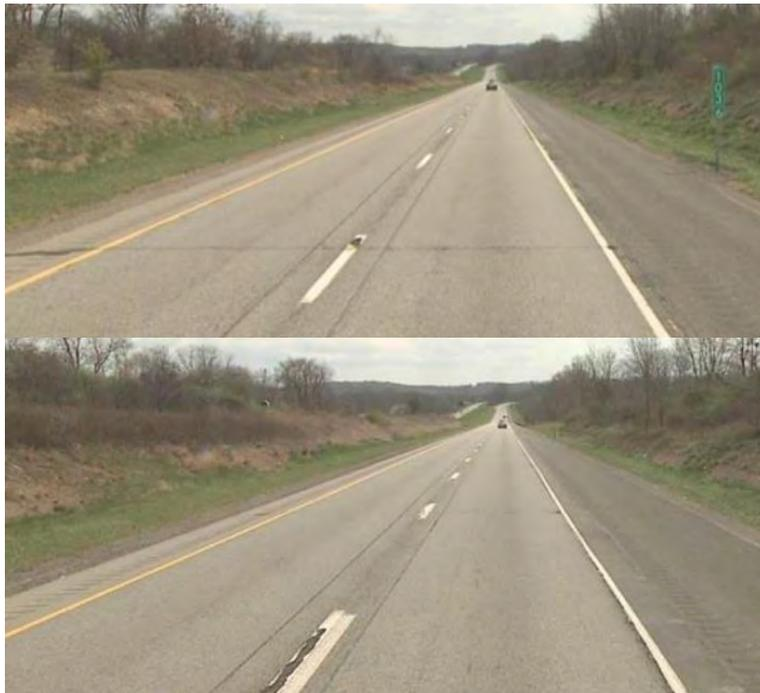
Figure 13: Pothole forming on I-79 skip lines
