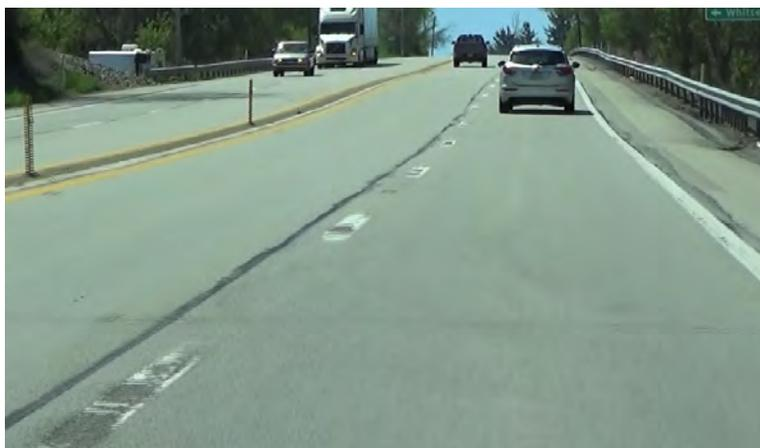
Figure 14: Asphalt raveling on PA-51 skip lines
