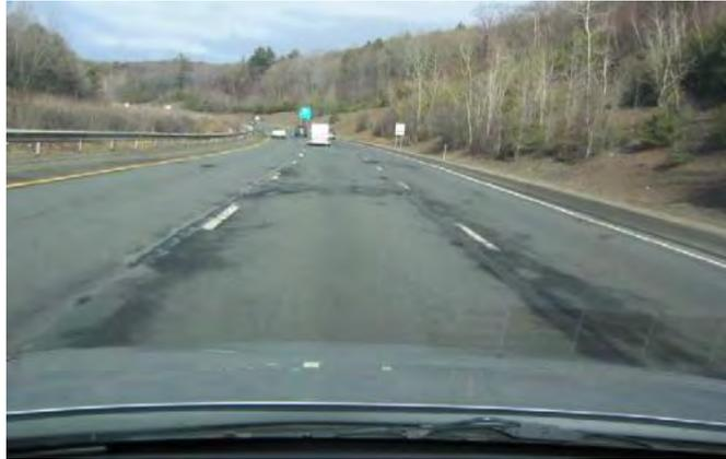
Figure 9: Deteriorated longitudinal joints with water infiltration [50]
