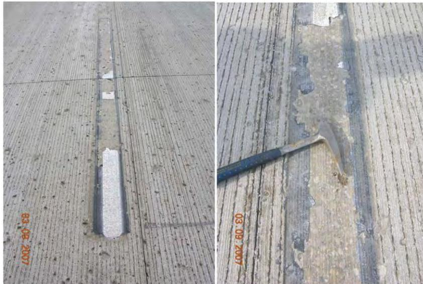
Figure 6: Missing or de-bonded pavement markings due to aggregate pop outs and poor bonding [19].
