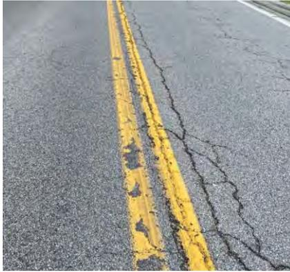
Figure 19: Centerline presenting cracking and losing marking material
