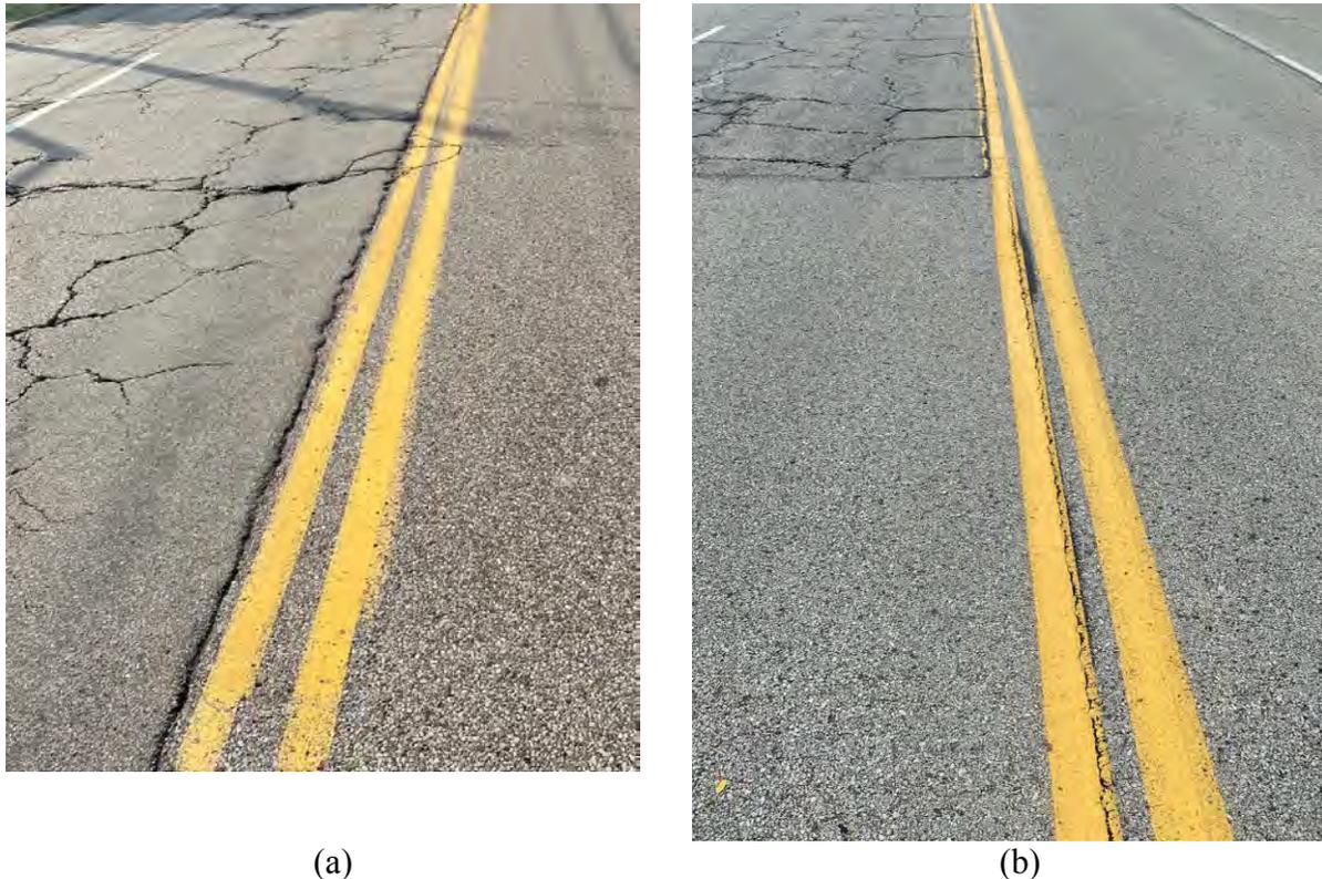
Figure 18: (a) Block cracking in two lanes with the centerline intact in the other lane and (b) longitudinal crack in only one of the centerline's lines
