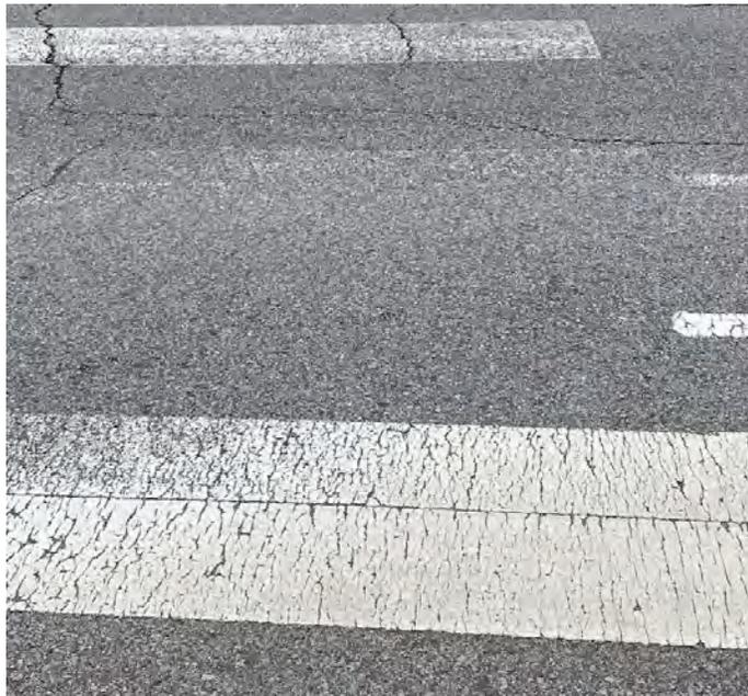
Figure 21: Pedestrian crossing markings with different levels of deterioration.
