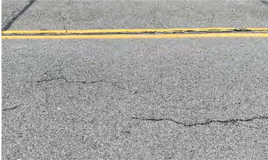
Figure 31: Pavement deterioration at the wheel path in Section 3
