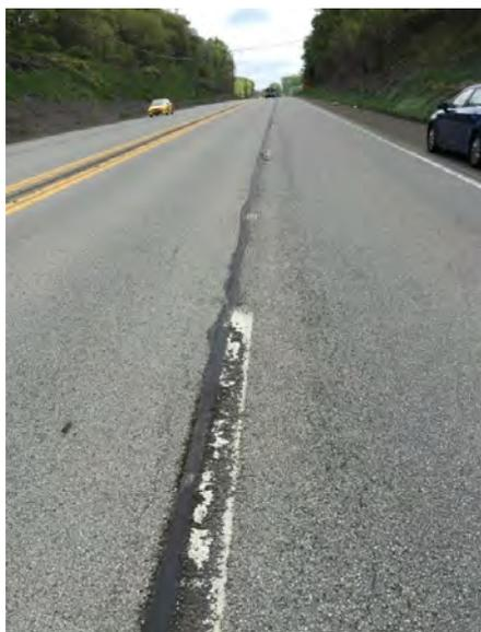
Figure 10: Surface delamination on US 422 skip line
