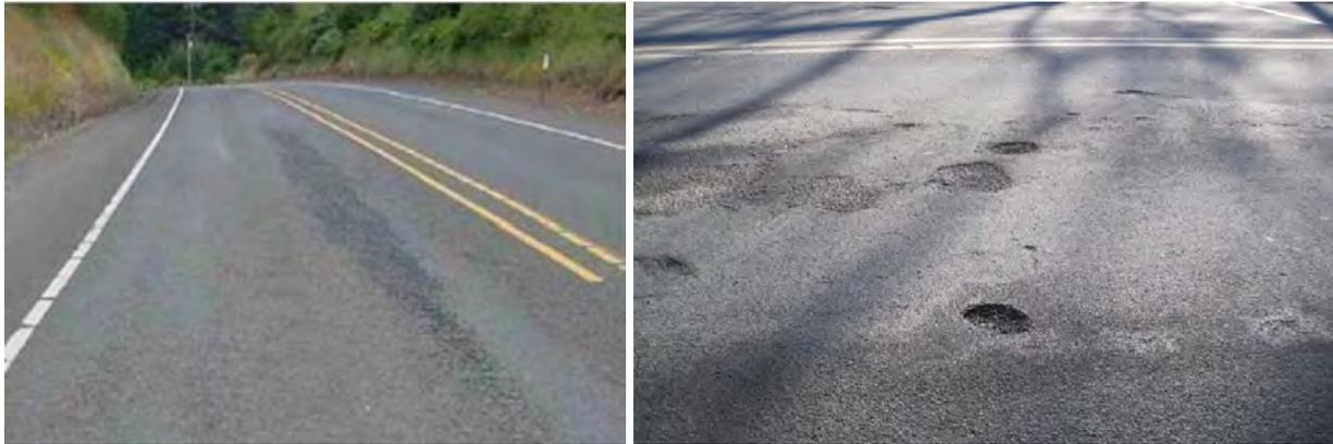
Figure 8: Raveling on asphalt pavement surface [27] and stripping between asphalt layers [28].
