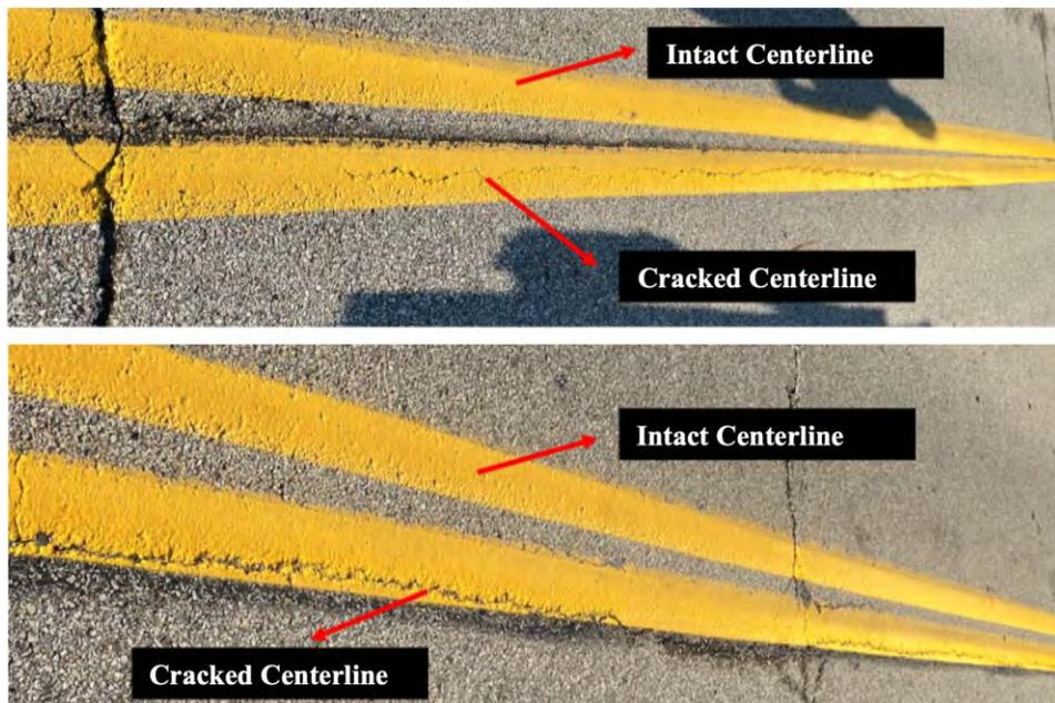
Figure 17: Examples of longitudinal crack in only one of the centerlines
