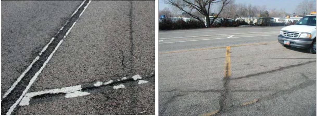
Figure 4: Pavement distress focused in pavement markings taken in Spring 2009 near Salt Lake City, Utah when the pavement was 7 years old with tape markings [18].
