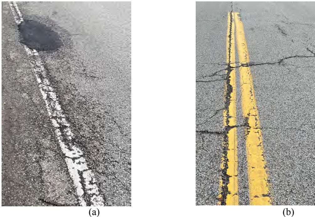
Figure 23: (a) cracking and potholes in the pavement shoulder joint and (b) cracking at the longitudinal joint
