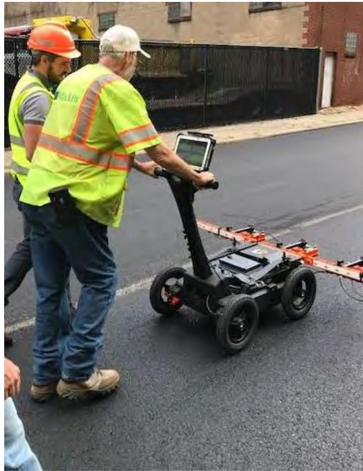
Figure 40: Density Profiling System (DPS) for real-time compaction assessment
