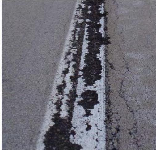
Figure 7: Pavement distress beneath polyurea pavement markings [13].
