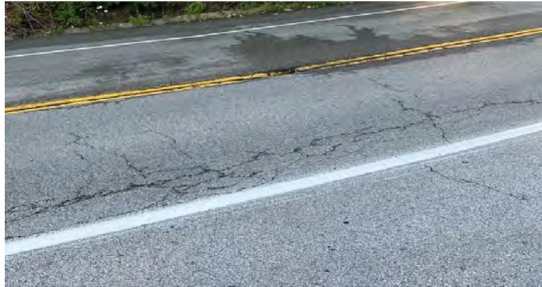
Figure 16: Cracking in pavement lane connecting to cracking in longitudinal joint
