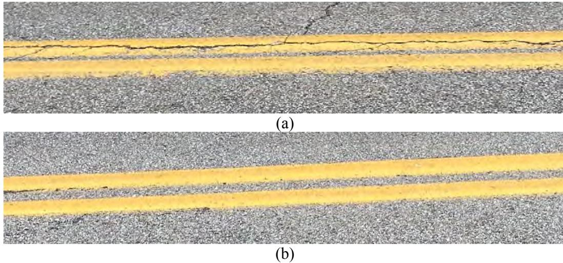
Figure 26: Segments presenting (a) deteriorated and (b) intact longitudinal joint area in Section 1
