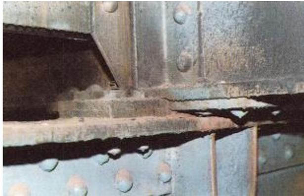
Figure 9. Fretting Corrosion at Stringer Joint [6]
