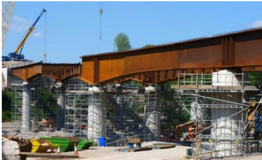
Figure 4. Bridge with Weathering Steel Girders [7]
