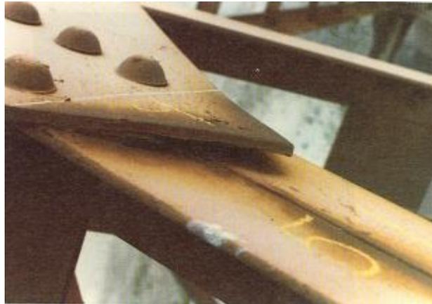
Figure 6. Crevice Corrosion, which has Caused Pack Rust and Bending Under a Gusset Plate [6]
