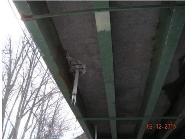
Figure 24 Improperly detailed free-falling scupper resulting in corrosion of bottom flange [41]
