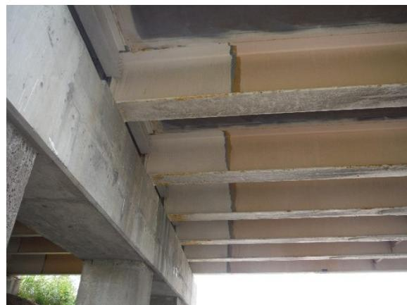
Figure 23 Polynox in girder ends of PA 136 Overpass over PA 51 after approximately 6 years of service
