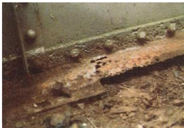
Figure 7. Pitting of Girder Web and Bottom Flange [6]
