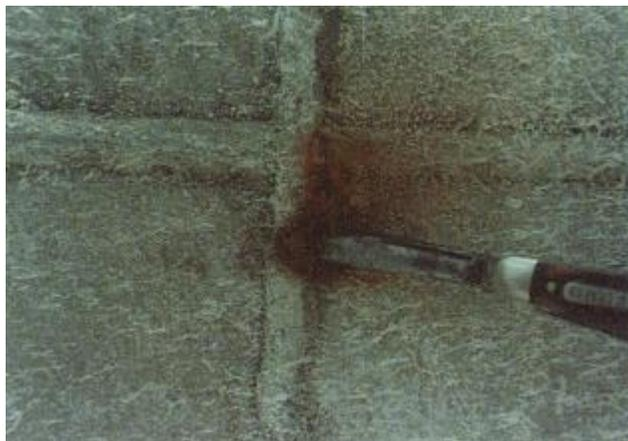
Figure 8. Weld Decay Corrosion [6]
