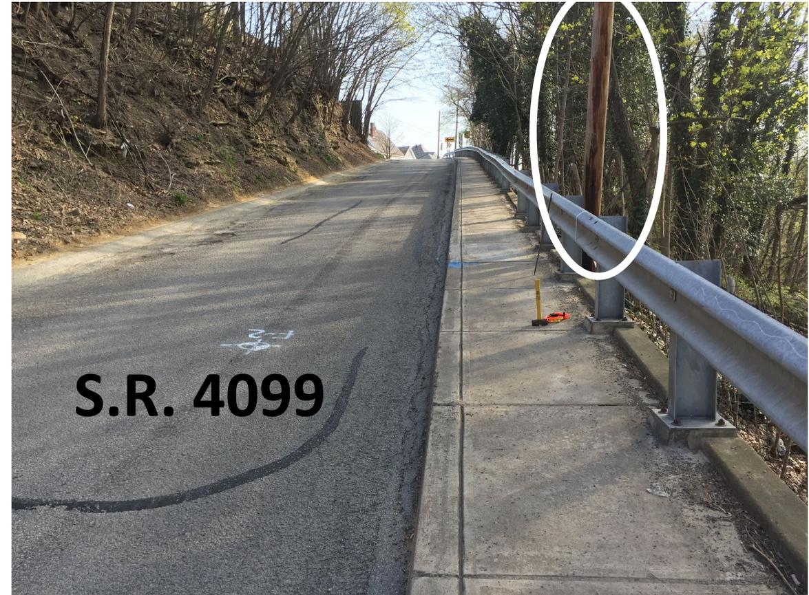
Sidewalk notch out for Pole #1, slope movement obvious
