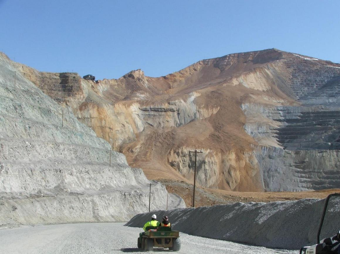
Instruments and radar detected critical wall movements. Pit evacuated prior to failure.
