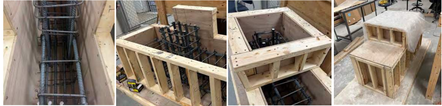
Conventionally Cast Reinforced Pier Cap
