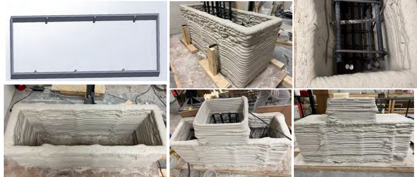
3DCP of Pier Cap Formwork
