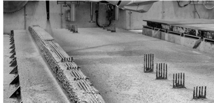
Concrete floor slabs with add-on-printed reinforced ribs
