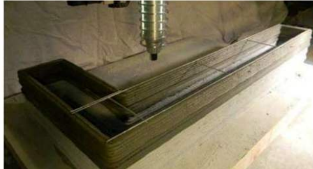
Placing steel reinforcement horizontally between 3d-printed concrete layers
