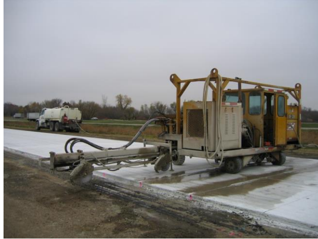
Figure 11. Sawing joints.
