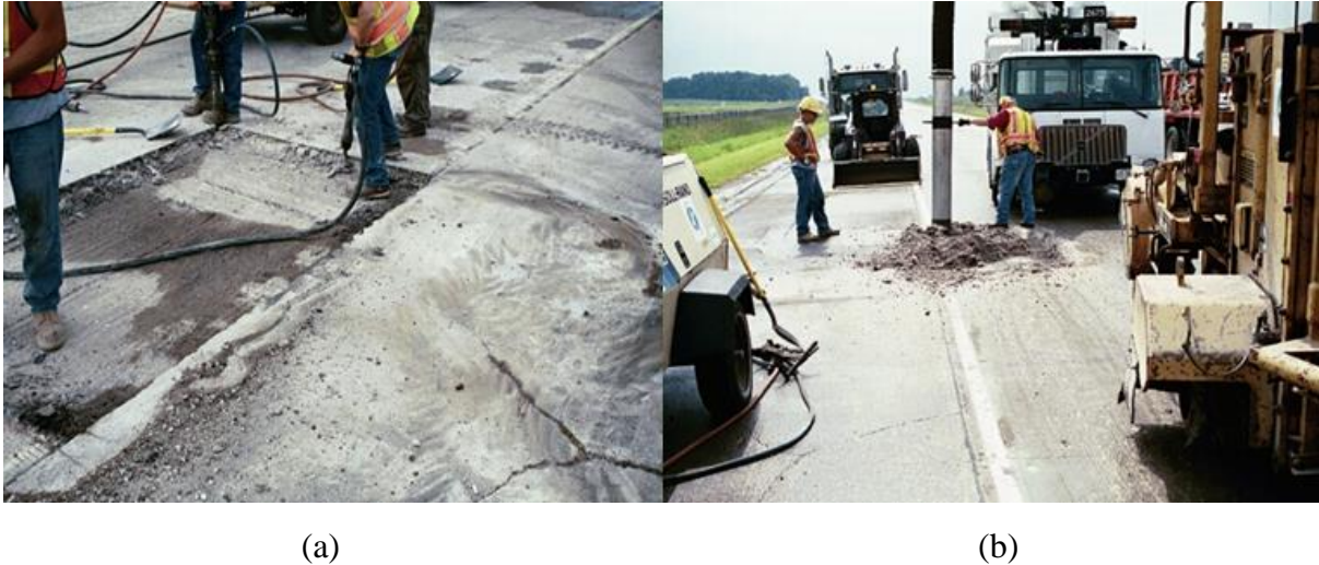
Figure 5. Material removal a.) jackhammering and removing the exterior edge and b.) removal of debris from the repair area.
