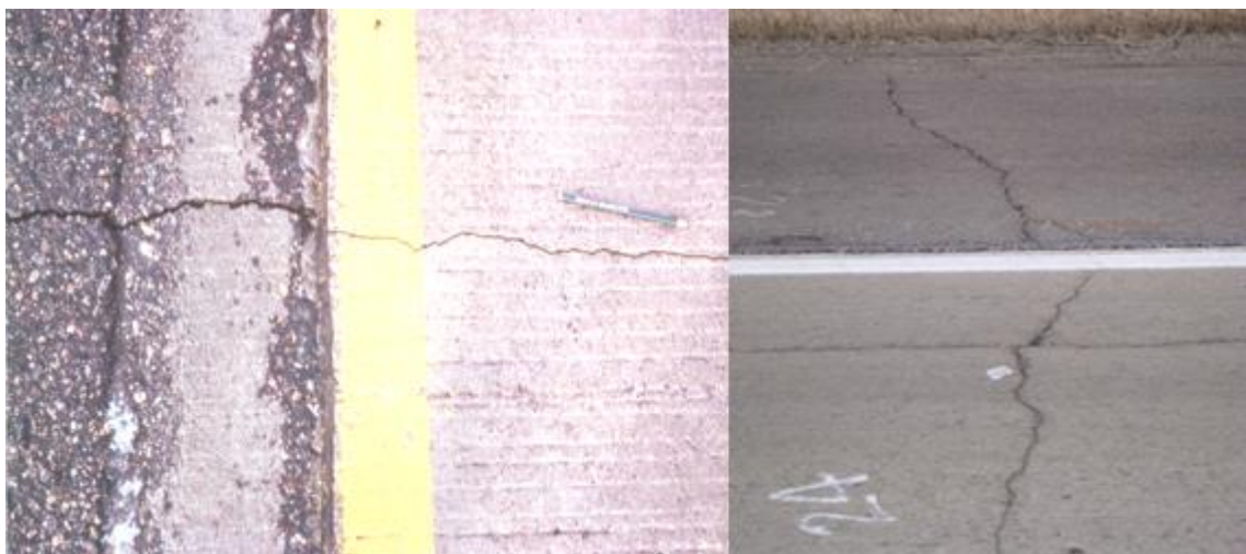
Figure 2. Reflective cracking in a BCOA.
