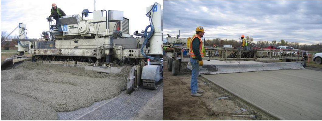
Figure 14. Paving and finishing an unbonded overlay.
