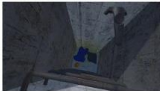
(e) confined space
