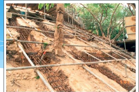
(a) Construction of soil nails and grillage.
