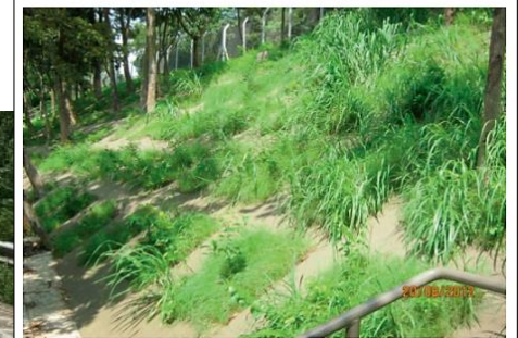
(b) Completion of soil nails and grillage construction.
