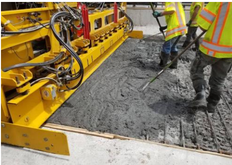
UHPC Overlay, Commodore Barry Bridge, PA&IA 2020
