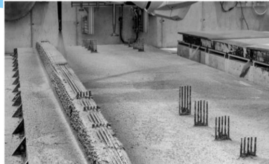
Concrete floor slabs with add-on-printed reinforced ribs
