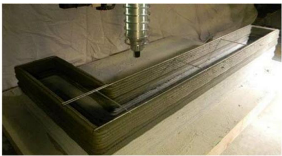
Place rebar while printing
