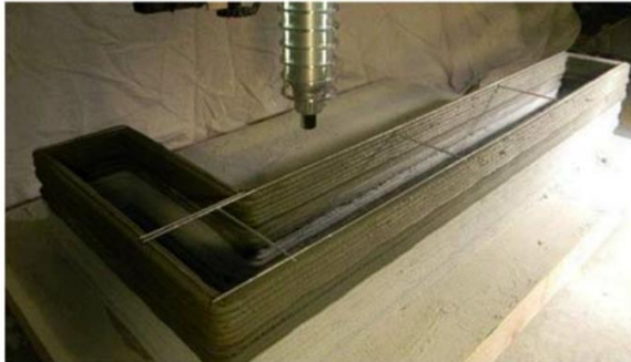
Placing steel reinforcement horizontally between 3d-printed concrete layers
