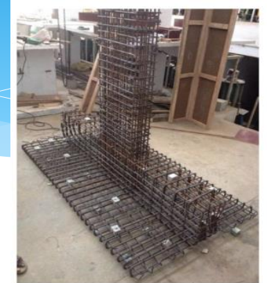
Double-loop twist ties is selected for typing rebar
