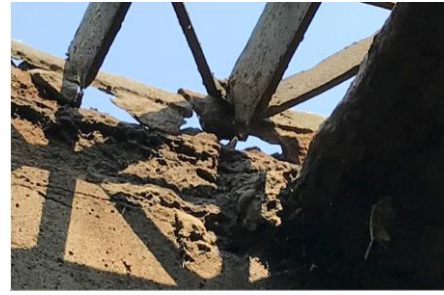
a) condition of far abutment prior to encasement (pre 2020)
