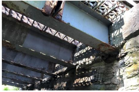
a) condition of far abutment prior to encasement (pre 2020)
