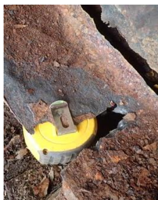
b) apparent cut through bottom flange
