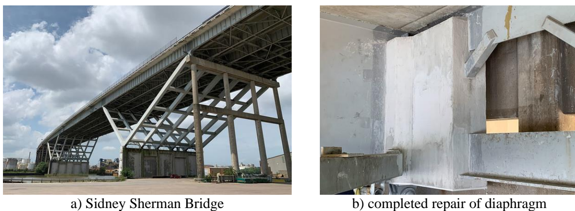
Figure 20 Field implementation of UHPC reported by TxDOT (2021)
