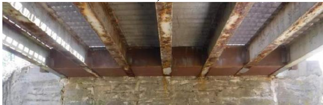
c) steel-formed concrete encasement at far abutment (post 2020)
