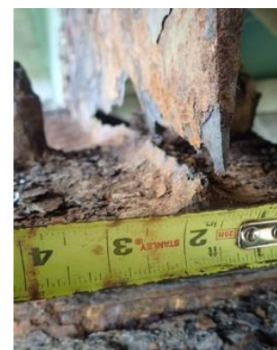
c) lateral distortion of web
