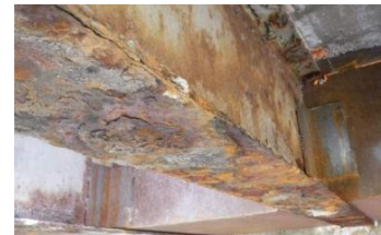
c) steel-formed concrete encasement at far abutment (post 2020)
