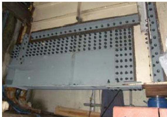
b) bolted beam end replacement (Wakabayashi et al. 2013) Figure 11 Steel beam end repair – replacing deteriorated region.
