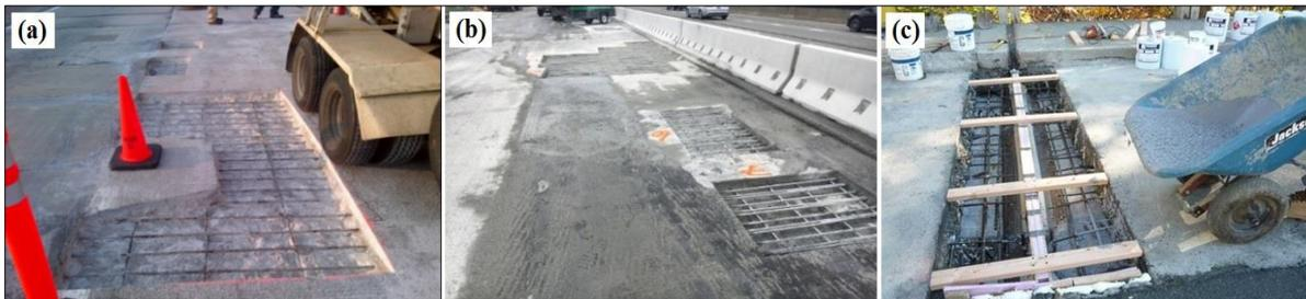
Figure 2. Concrete bridge deck repair types. a) Deteriorated concrete extends to the depth of top of the reinforcing bars, b) Deteriorated concrete extends beyond the depth of top of the reinforcing bars, c) Deteriorated concrete extends to the full depth of the deck [2], [3]
