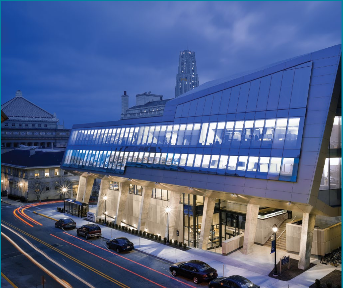
Benedum Hall houses Pitt's Swanson School of Engineering.
